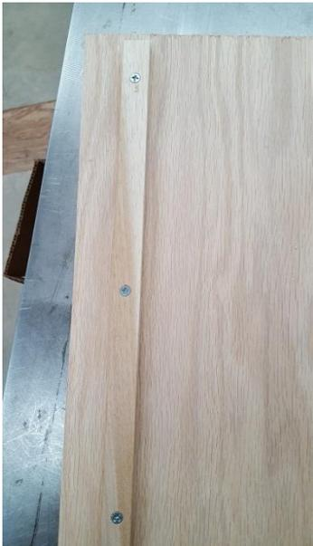
After the glue sets turn upside down and screw the runners into the board.
